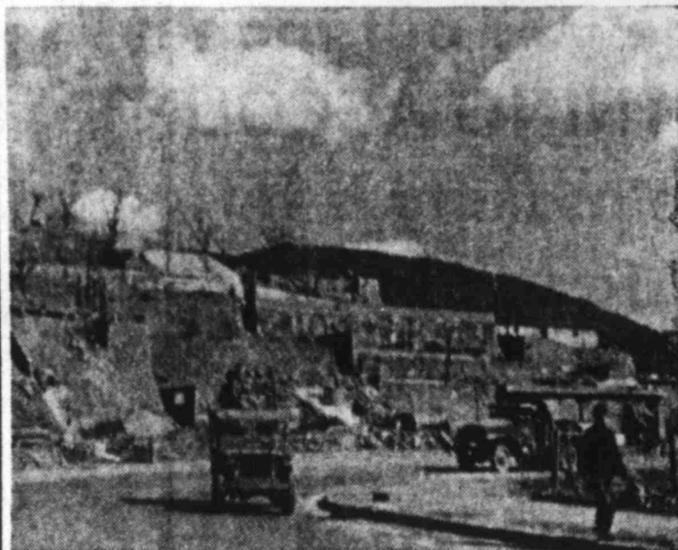
Just foundations going up the hill, no houses...
