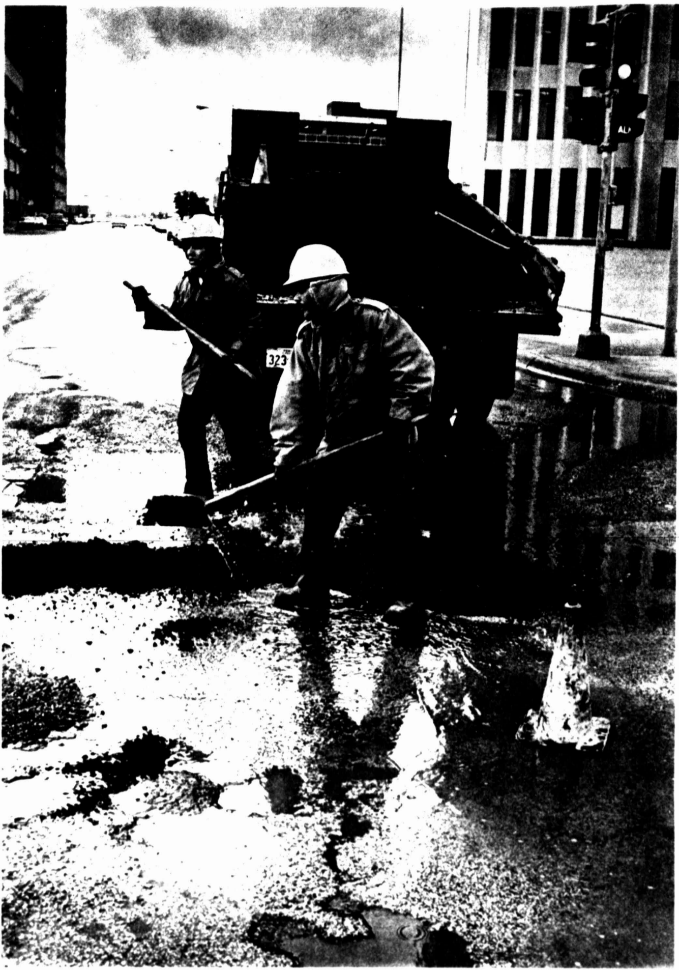
Puddles from this morning's rains afford city workers Noah Martinez, left, and Placido Sifuentes an opportunity to see which chuck holes at the corner of Illinois Avenue and Marienfeld Street need filling the worst. (Staff Photo)
