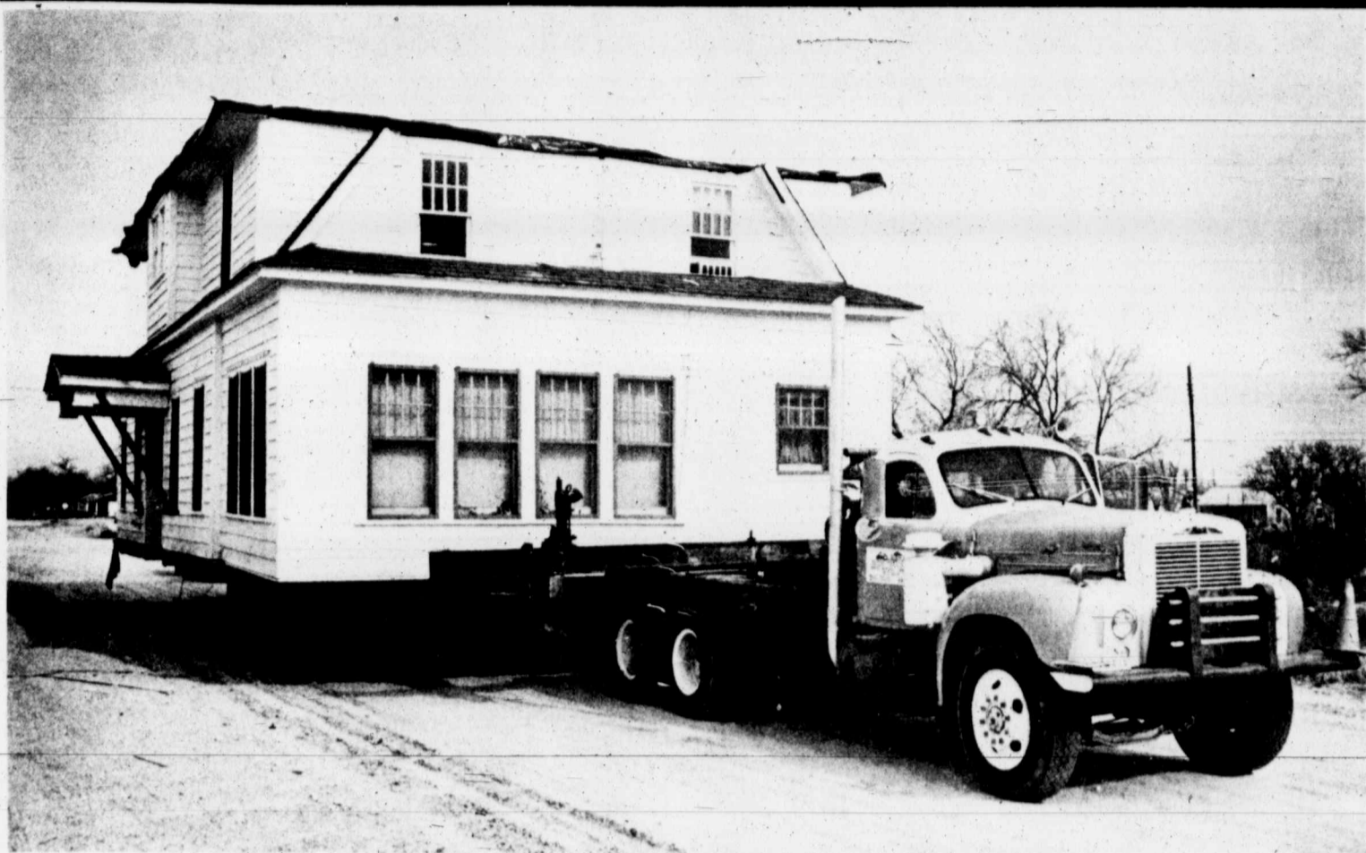
Instead of a family going to its new house, this house — which isn't new — moves to the Terry Dossey family. Weighing in at about 110,000 pounds, the two-story house was transported Wednesday from 211 W. Kansas
