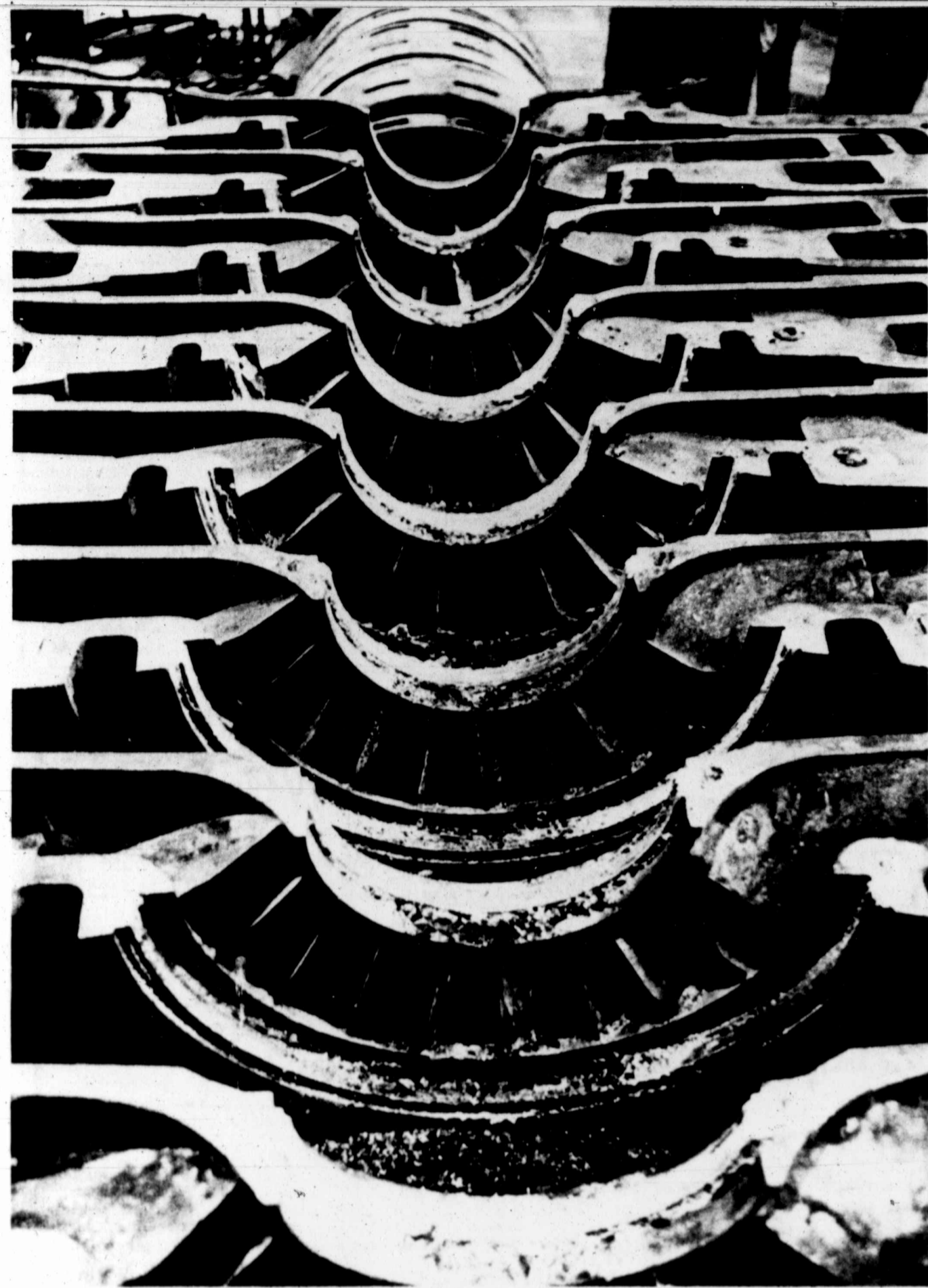
Can you guess what this is? No, it's not a row of pipe organs, a stack of false teeth or a line of pigeonhole desk slots. It's the inside of a 30-ton gas compressor going through routine maintenance and repairs at Amoco-Texas Refining Co.'s oil refinery in Texas City.
