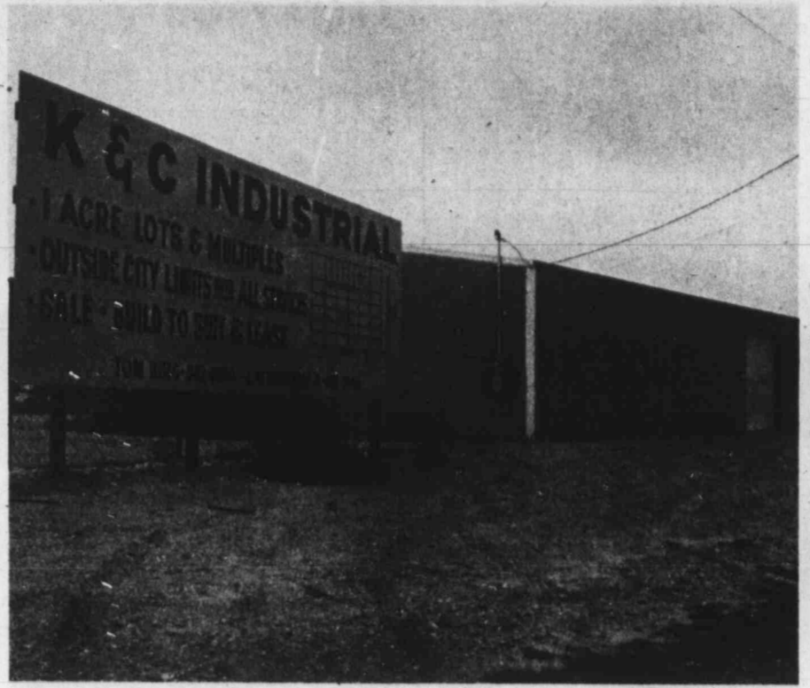
Show is one of the warehouses in K&C Industrial's new planned district. Located on Francis Avenue west of Cotton Flat Road, this new development features modular space units, metal or tilt-wall buildings suitable for warehouses and shops for light or heavy manufacturing. Call Tom King or Sookie Harward at 682-6000, or Bill Chancellor, 683-2040.
