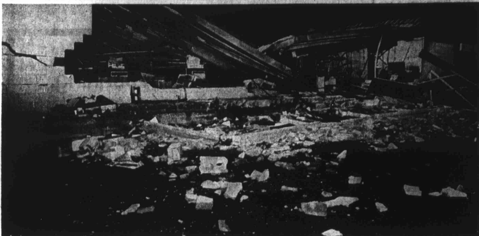
FATAL FIRE — Two Lubbock men were killed about 1 a.m. today when an explosion rocked this convenience store at 704 E. Broadway. The owner of the building, Andrew Zournas, 52, of 3011 42nd St. and Mark Corley, thought to be in his 30s, of 2126 52nd St. were pronounced dead at the scene. Firemen fought the resulting fire about 1½ hours. The deaths brought Lubbock's 1979 fire-related toll to three. (Staff Photo by Paul Moseley)
