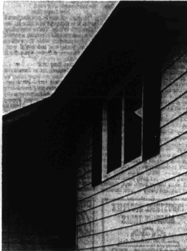
FOR FUNCTIONAL BEAUTY — United States Steel siding, soffit and fascia systems are the specialty of Gill Construction Co., now at its new 4901 Brownfield Highway location in Lubbock.
