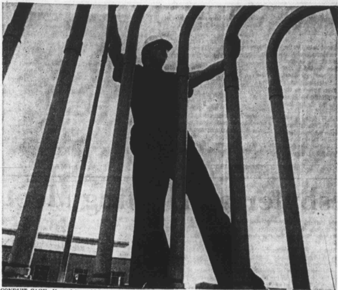
CONDUIT CAGE—If conduit could be compared to bars, it might be said that Buck Barnard of La Porte appears to be imprisoned as he makes a routine equipment inspection. The pipe cage is actually part of a Tenneco Oil Co. fractionating plant near Houston. Added demand for petroleum products has required increased output from such facilities.
