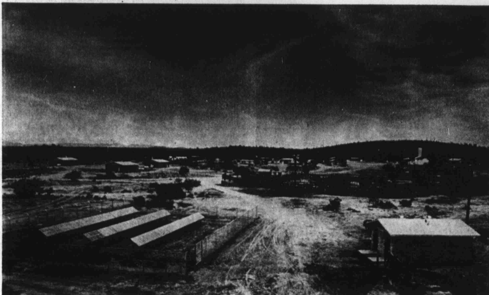
SOLAR VILLAGE—This 3,500-watt solar cell array field, shown at left, is the main element of the world's first solar electric village power system. The system is designed to provide sufficient electricity to meet the basic energy needs of the 96 residents of
