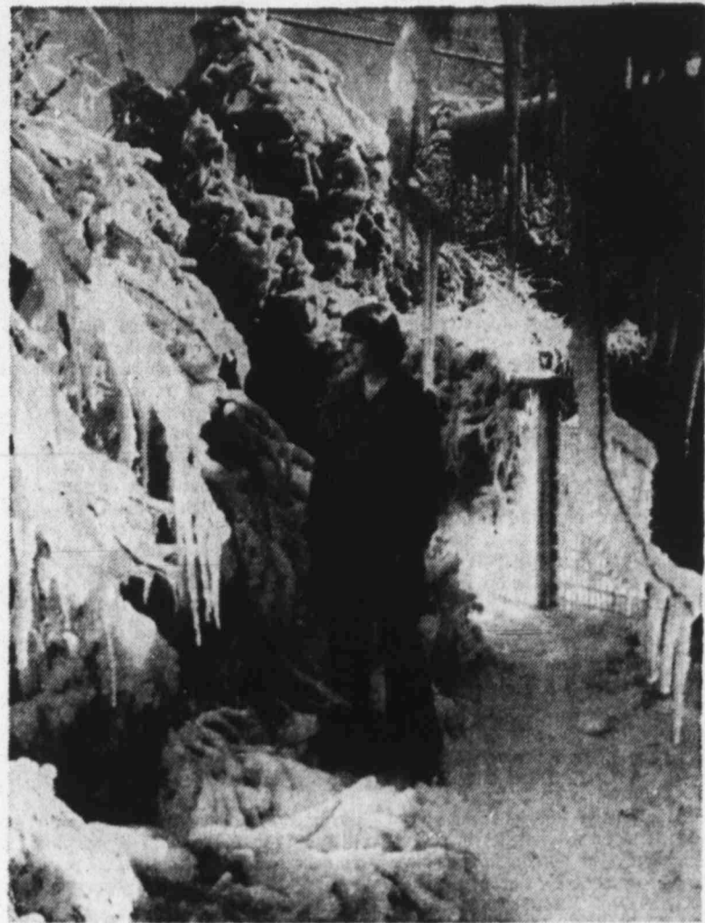
ARTIFICIAL WONDERLAND — Mrs. Mike Weinman of Tulsa, Okla., views consequences of a pre-dawn water leak which encased her house and surrounding trees with ice. Tulsa water crews eventually shut off the geyser, which erupted as 11-degree temperatures hit this week. (AP Laserphoto)
