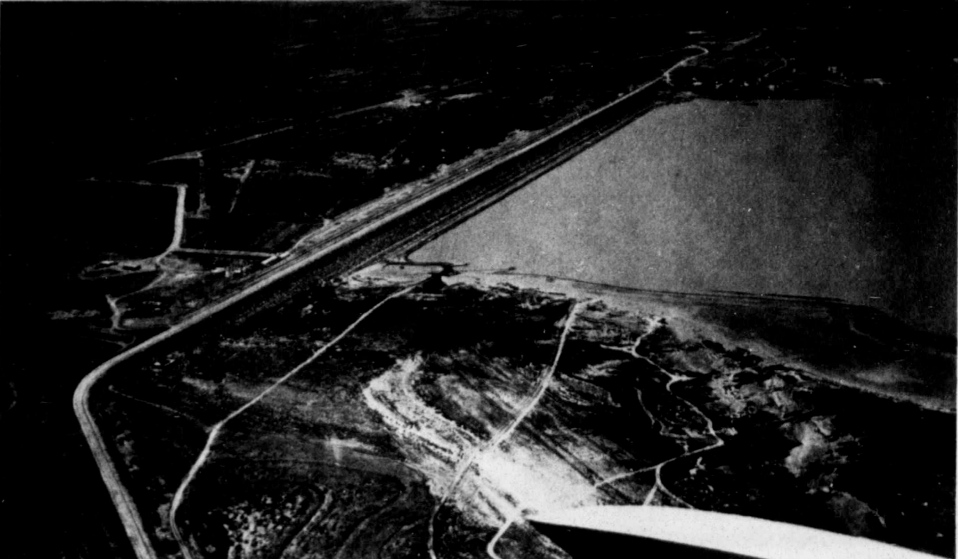
The declining water level of Lake J.B. Thomas in Scurry and Borden Counties was a consideration eight years ago when the Colorado River Municipal Water District initiated a weather modification program.
