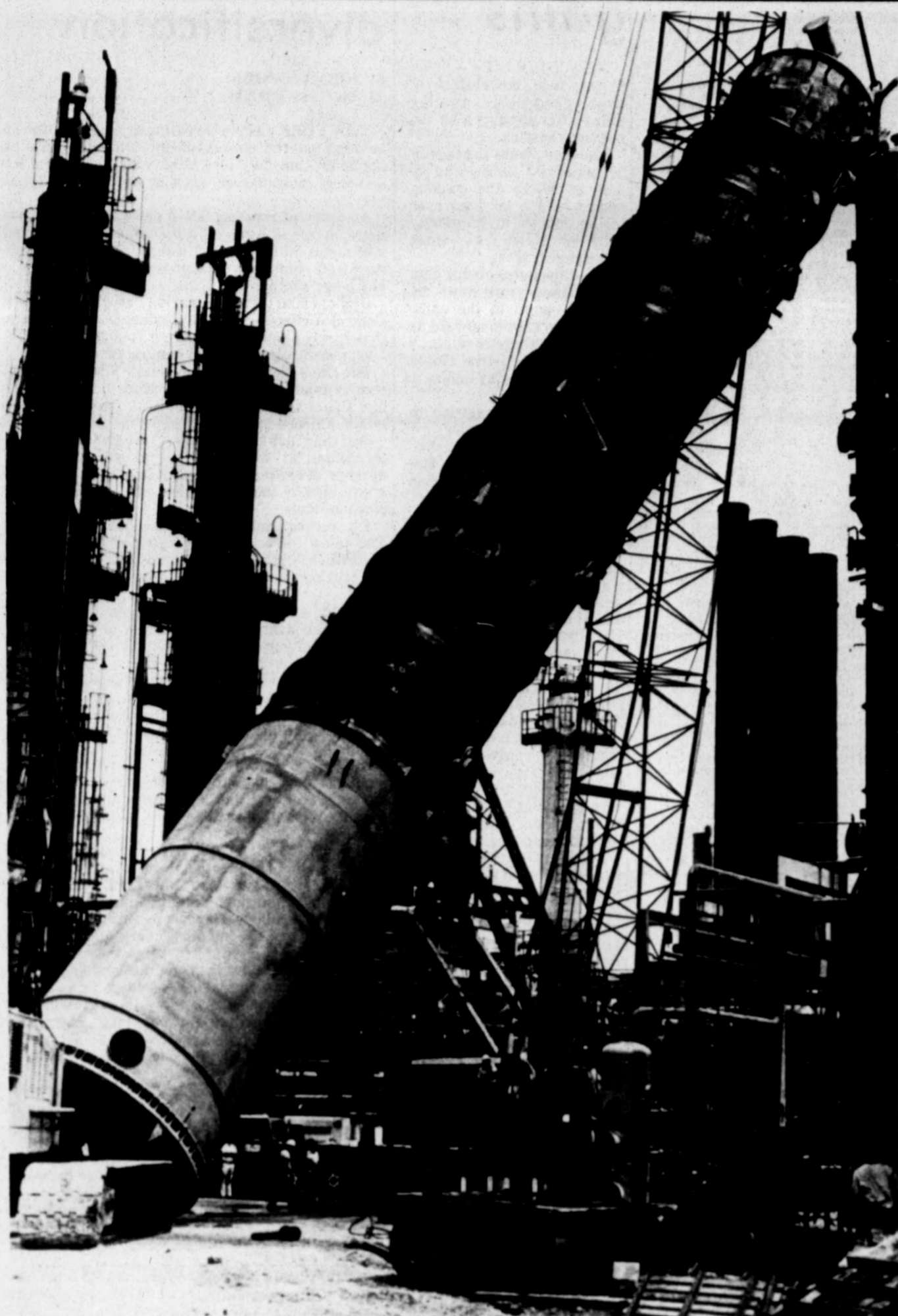
This gas oil fractionator is representative of the enormous pieces of equipment required at Amoco Texas Refining Co.'s oil refinery in Texas City. Weighing 180,000 pounds and measuring 130 feet
