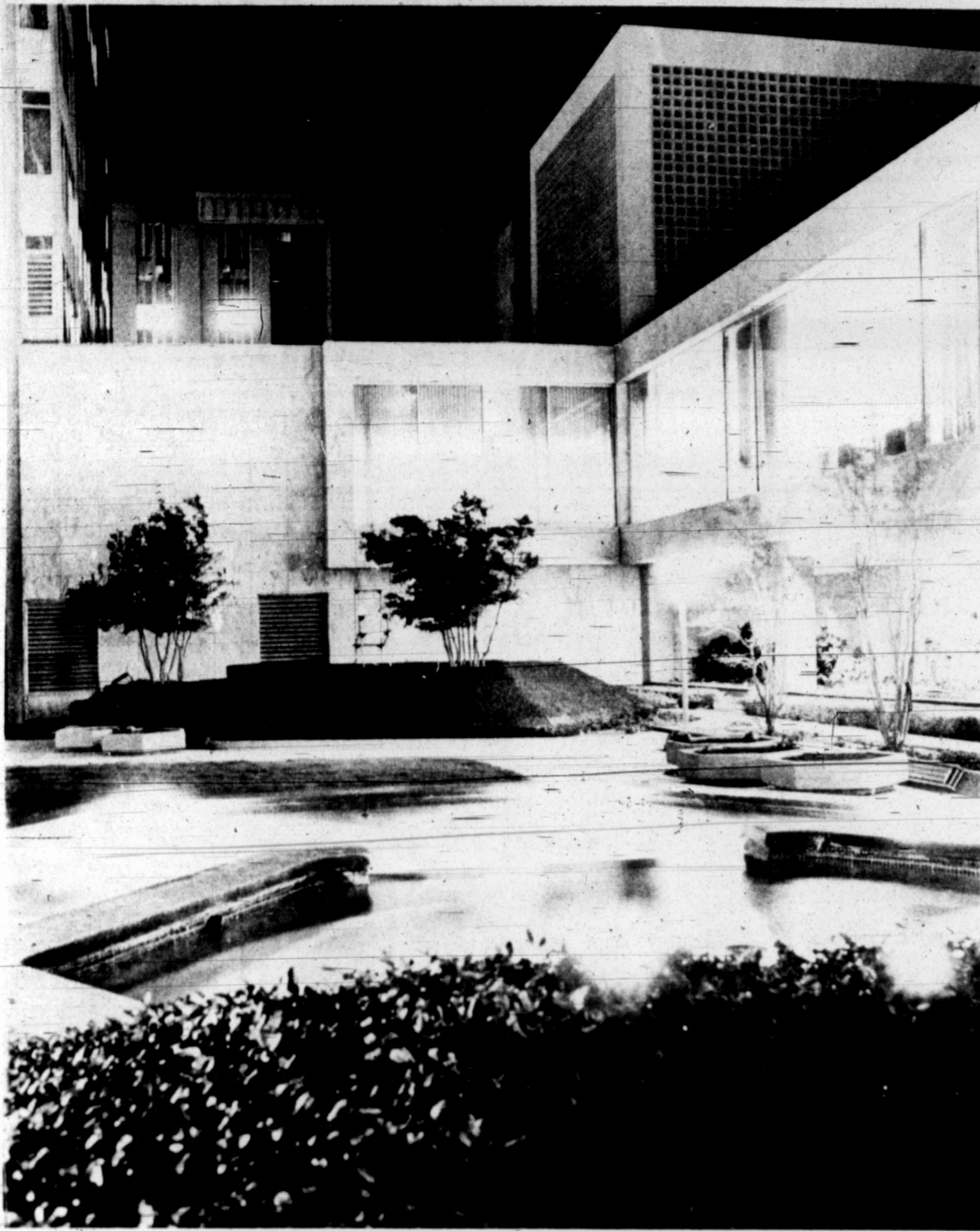
Part of The First National Bank of Midland's beauty can be found in this plaza situated on the northwest corner of the bank's downtown property. The plaza was inspired by C. J. Kelly, former bank chairman and now an honorary member of the board. Jim Stephenson, vice president and
