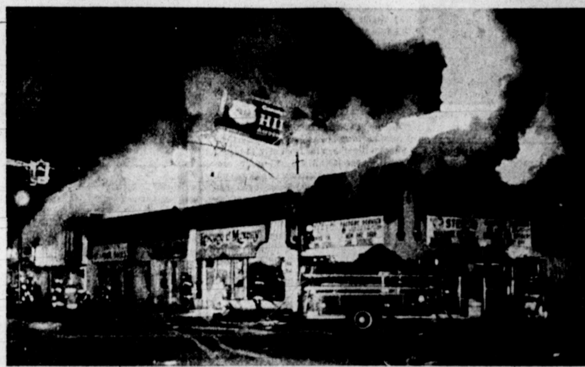
EARLY MORNING FIRE — This was the scene near downtown Dallas today when fire broke out and consumed several businesses in a shopping mall. There were no injuries reported and a damage estimate had not been given. (AP Laserphoto)
