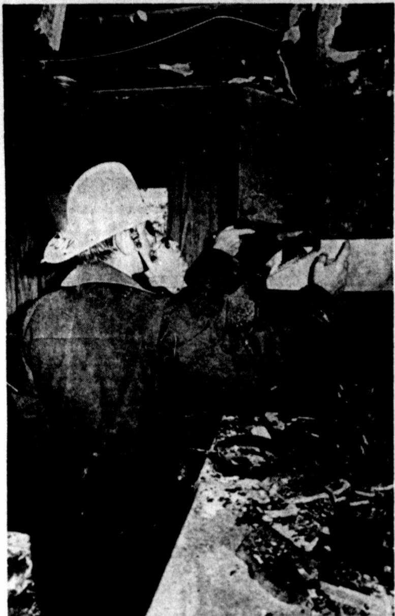
CHECKING OUT THE CAUSE — Lt. Don Hart, in hat, and acting District Chief Les Hooper check the area around an apparent malfunctioning electric stove which caused more than $1,000 damage to a unit in the Sunset Apartments at 5801 22nd St. Saturday afternoon. Four units were called to the scene and firemen were able to contain the fire to the one apartment occupied by Jerry Carmichael, who was not home at the time of the blaze. (Staff Photo)
