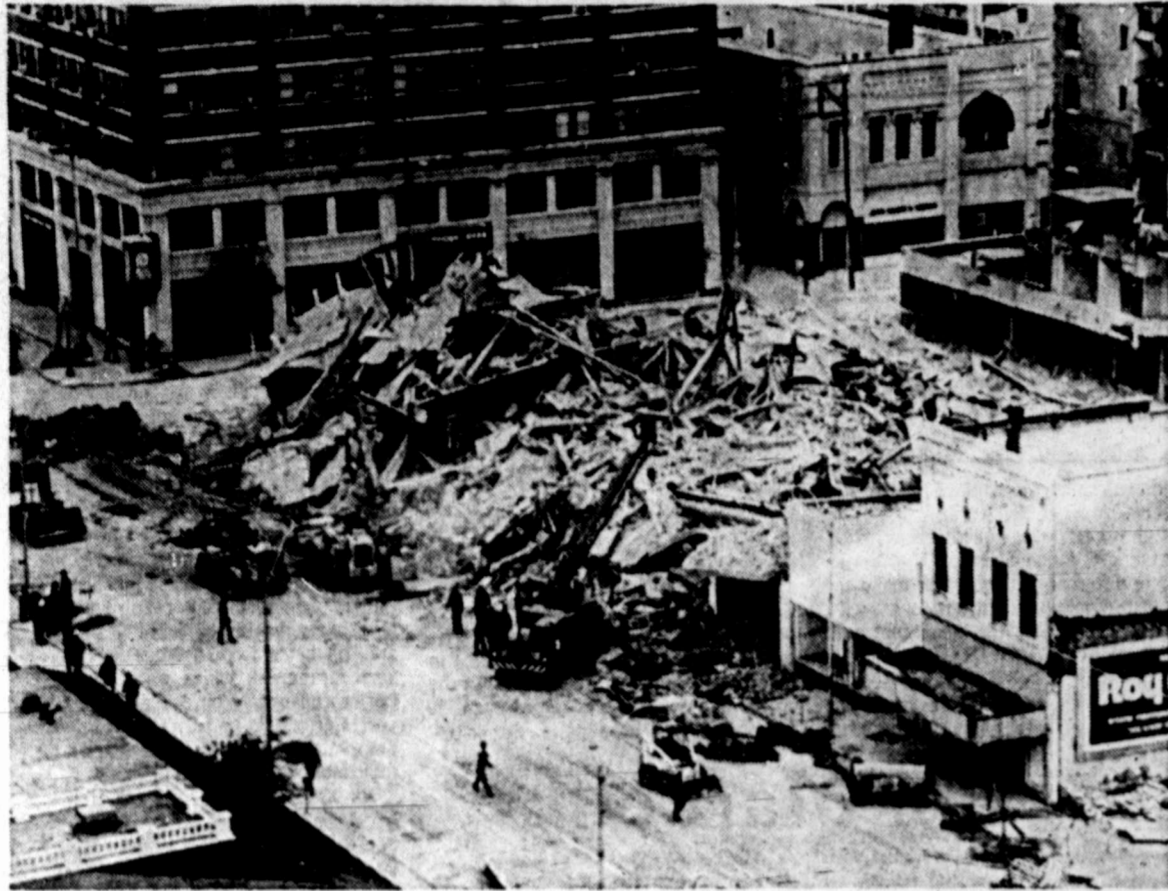
BUILDING COLLAPSE — Workmen seek to remove rubble of a Joplin, Mo., hotel which collapsed Saturday, burying a number of workmen. Rescue efforts were continuing through the night. (AP Laserphoto)
