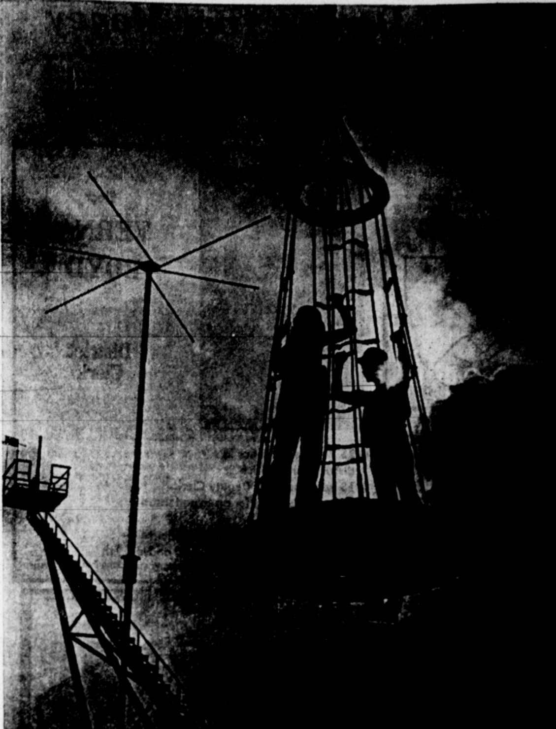
OPEN AIR ELEVATOR —It's nothing like one would find in a fancy office building, but this elevator gets the job done on a Tenneco Oil Co. drilling and production platform in the West Cameron area of the Gulf of Mexico. While it is a long way from the water line to the upper reaches of the platform, this airborne basket makes the trip quickly. And with a backdrop of sun and clouds, the scene takes on an aspect of art.
