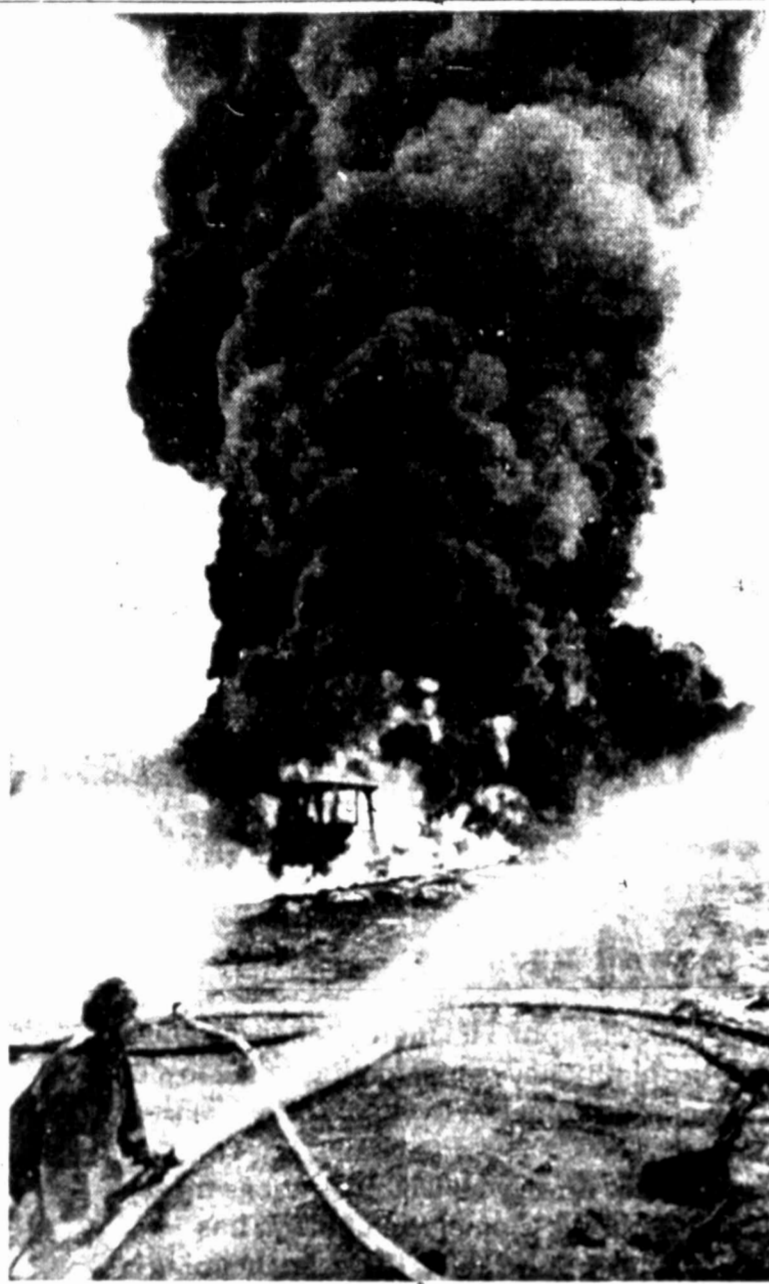
OIL PIPELINE FIRE—A Corsicana fireman pours water on oil pipeline fire Tuesday near Corsicana. The pipeline was broken and ignited when a bulldozer plowed up a section of the line...
