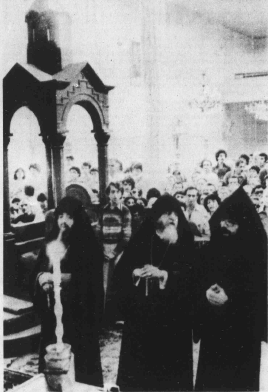
Khoren I, center of the Orthodox Armenian Church of Cilicia, center, and his Coajutor Karekine II, formerly of New York City, right, pray for dead and wounded congregation members at 40 Saints Church in East Beirut's Bourj Hamoud district Tuesday. The hole in ceiling, top center, is one of many in the church which was caught in the artillery and rocket duels between Christian rightist militias and Syrian troops of the Arab peacekeeping forces during the past nine days. (AP Laserphoto)
