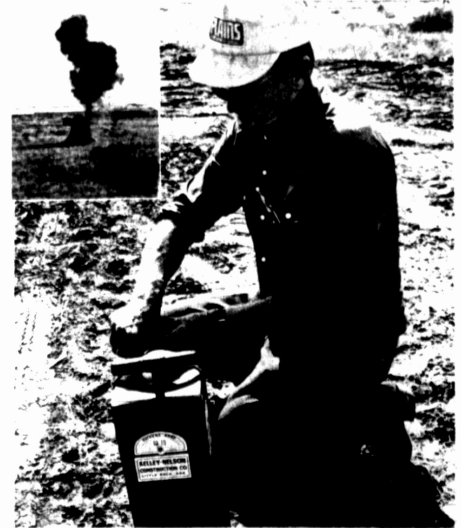
Myrl Anderson of Odessa connects the detonator for one of six charges set off Tuesday in groundbreaking observances for Midland Mall. A small puff of smoke and a blast of noise resulted from each of his efforts, as intended. (Staff Photo)
