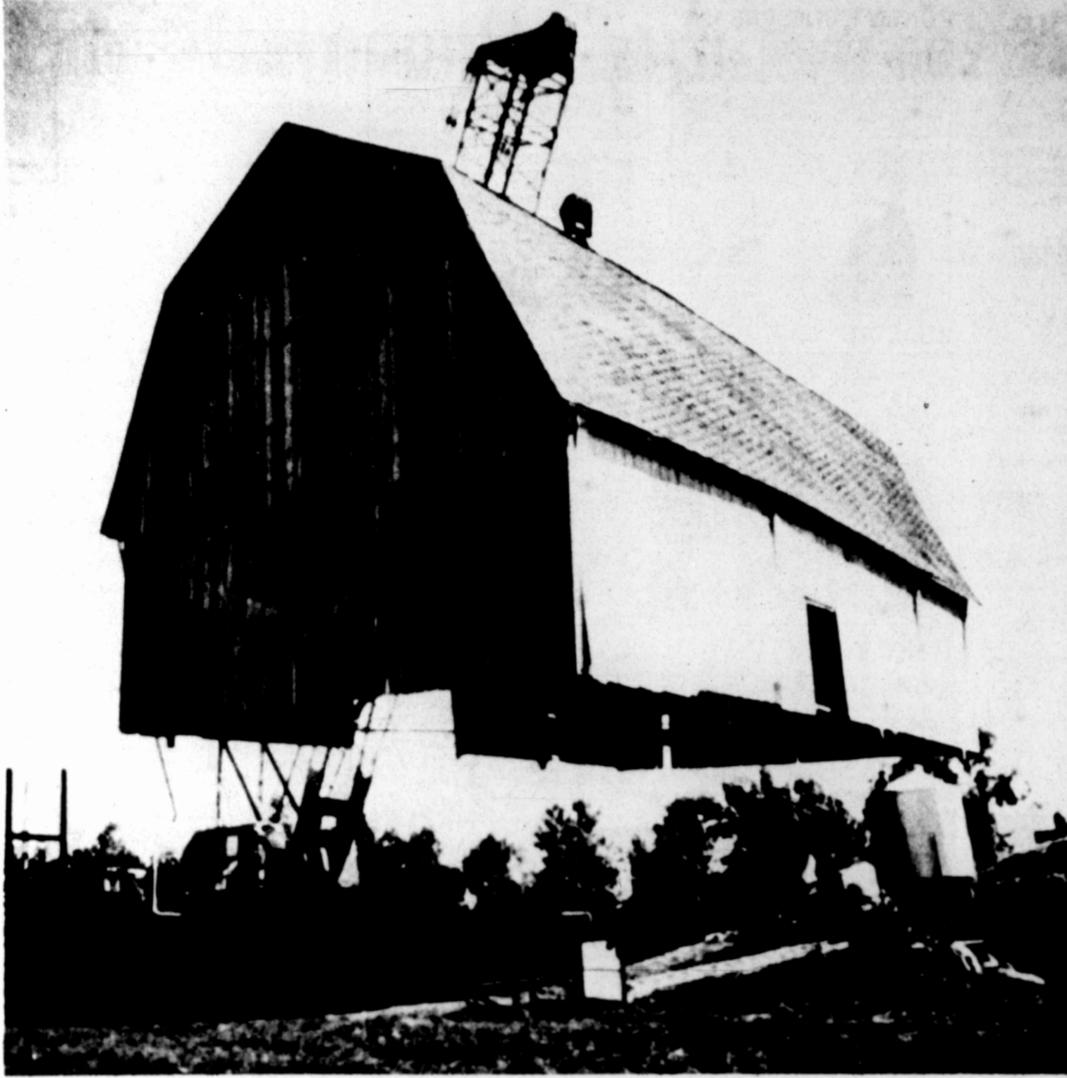
THE FOUNDATION of B.A. Dammen's 100-year-old barn was collapsing, so he decided to give it a lift. He built a new foundation for it on his farm near St. Clair, Mich., and hired a crane company to make the move. The 110-ton crane picked up the barn and moved it 100 yards without a mishap. Cost of moving the barn was less than building a new one, Dammen said. (AP Laserphoto)
