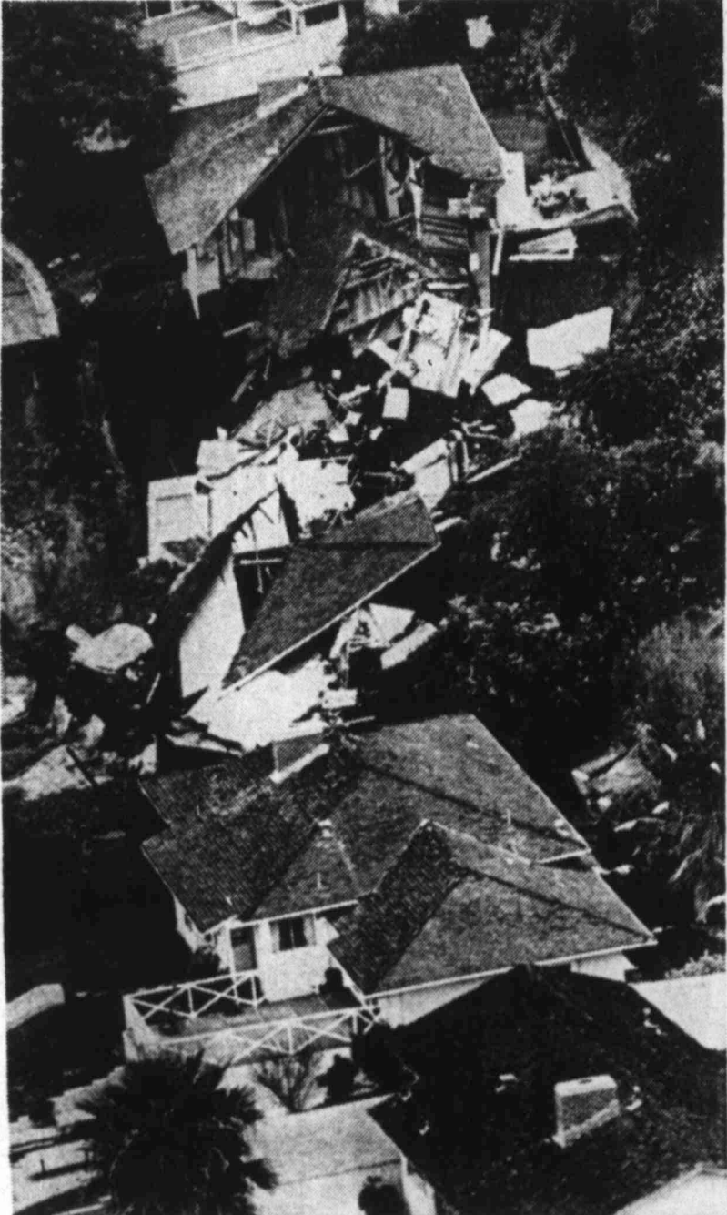
SLIDE DAMAGE HEAVY — This aerial view of some of the homes caught in the landslides at Laguna Beach, Calif., shows the heavy damage to the area. Scores of residents had to be evacuated because of the loss of their homes and the disruption of sewer, water and phone service. (AP Laserphoto)
