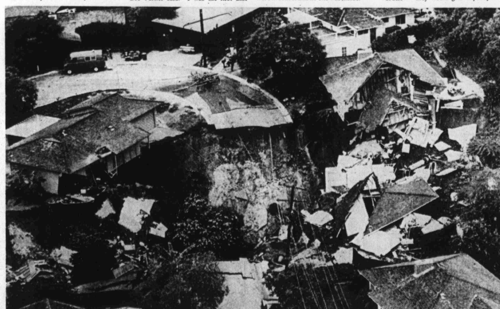
HOMES DESTROYED BY SLIDES — The awesome devastation caused by landslides in this fashionable area of Laguna Beach, Calif., is shown in this aerial photo. At least 49 of the expensive residences are destroyed or severely damaged, forcing the evacuation of about 200 persons. (AP Laserphoto)
