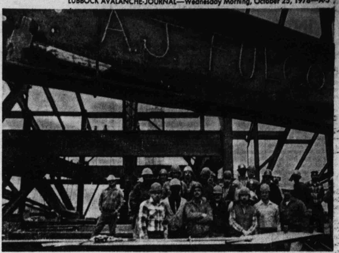
PAYING TRIBUTE — Ironworkers gathered Tuesday under a beam which will serve as a memorial to A. J. Fulco in the structure of the Federated Department Stores office building in downtown Cincinnati. Fulco fell to his death from the structure
