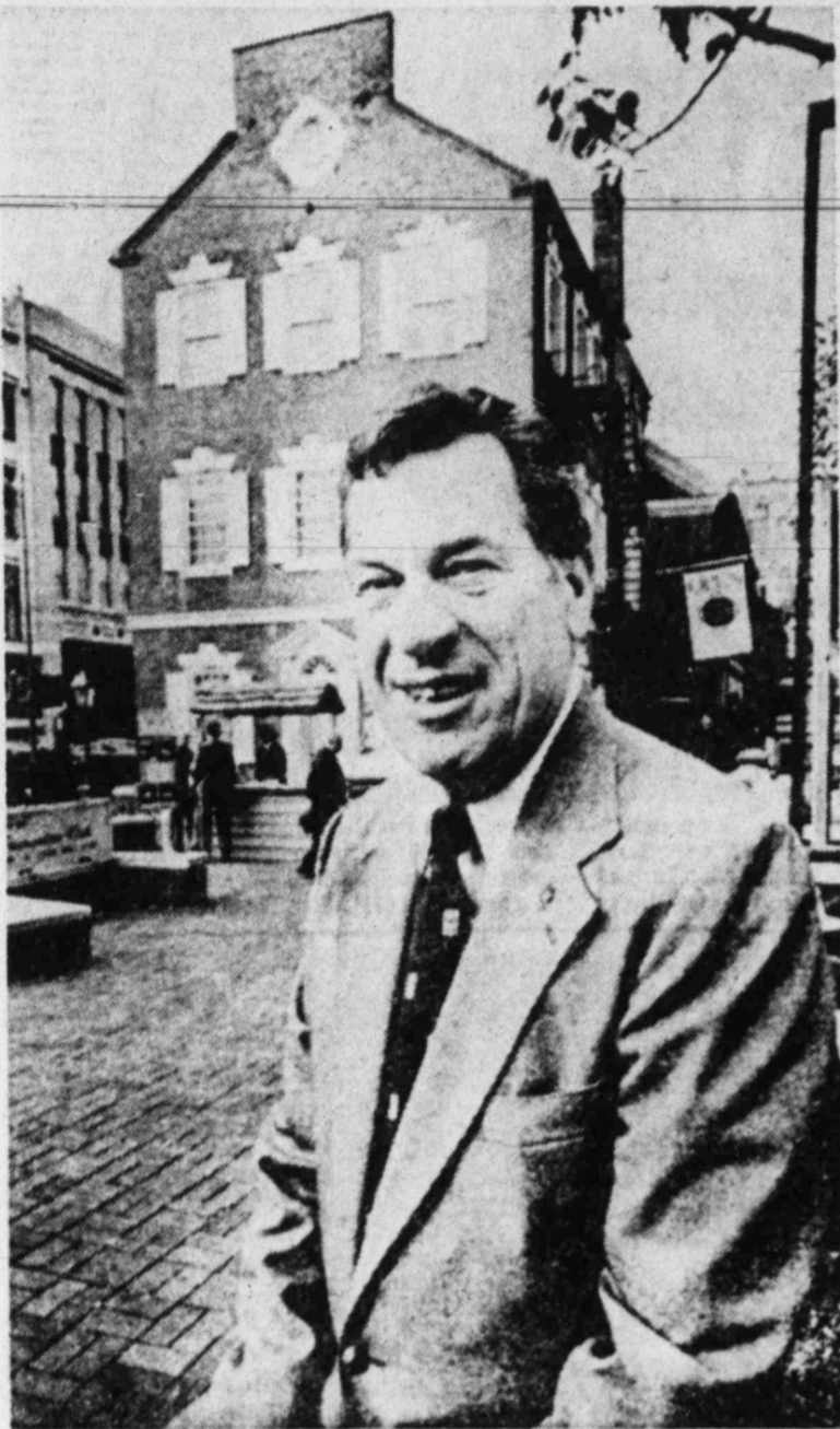
LANCASTER RESTORATION — Mayor Richard M. Scott stands in front of Old City Hall, which is undergoing restoration, in Lancaster, Pa. Lancaster is in the heart of Amish country, where the benefit of progress has long been questioned but renovation has brought back to this city its old vitality. (AP Laserphoto)
