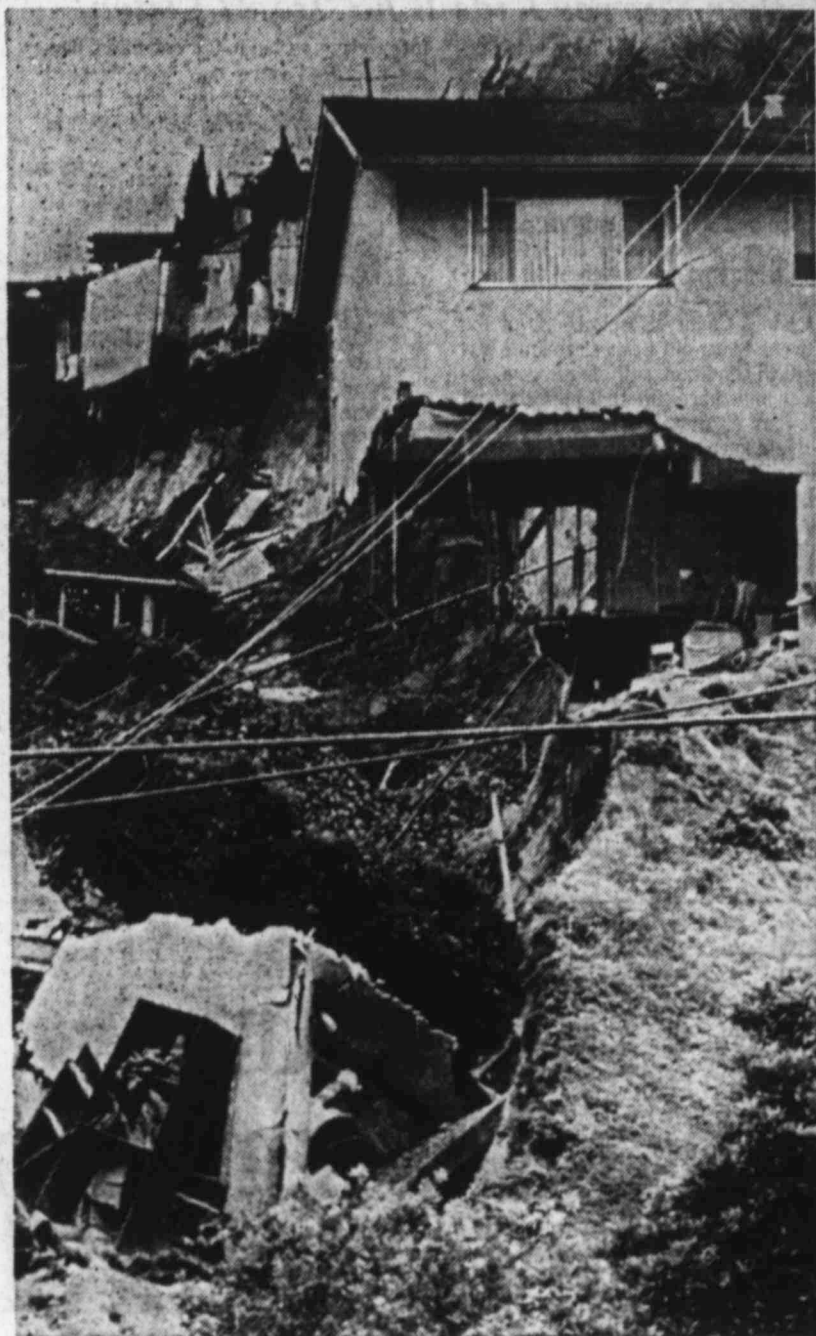
LANDSLIDE AFTERMATH—Shown in the left panel are the remains of four of the homes lost to a landslide in Laguna Beach, Calif., Monday. At least 49 homes were destroyed or badly damaged. Power, water and gas lines were ruptured, but there were
