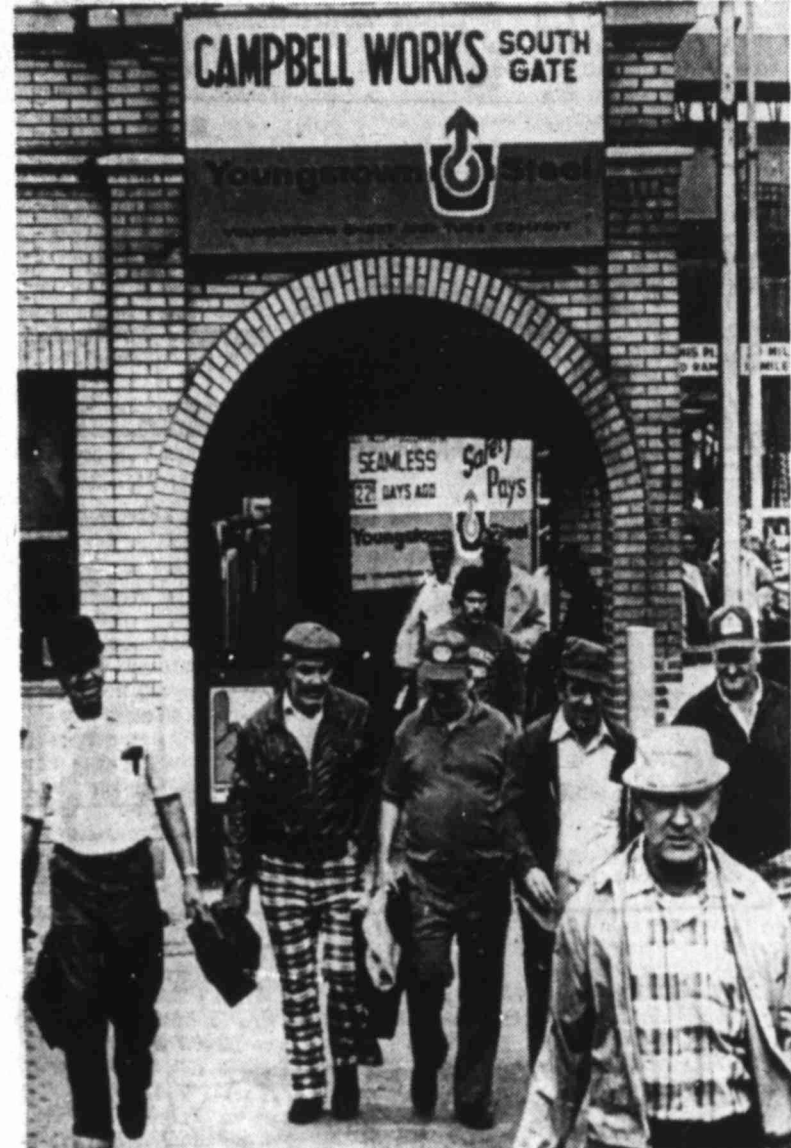
LEAVING BEHIND BETTER DAYS — Steelworkers leave the Youngstown Sheet & Tube Co.'s Campbell Works in Campbell, Ohio, a Youngstown suburb, prior to the aging facility's closing a year ago. In a town where 75 percent of the municipal income came from the mill, shock waves from the closing are still being felt in the community. (AP Laserphoto)
