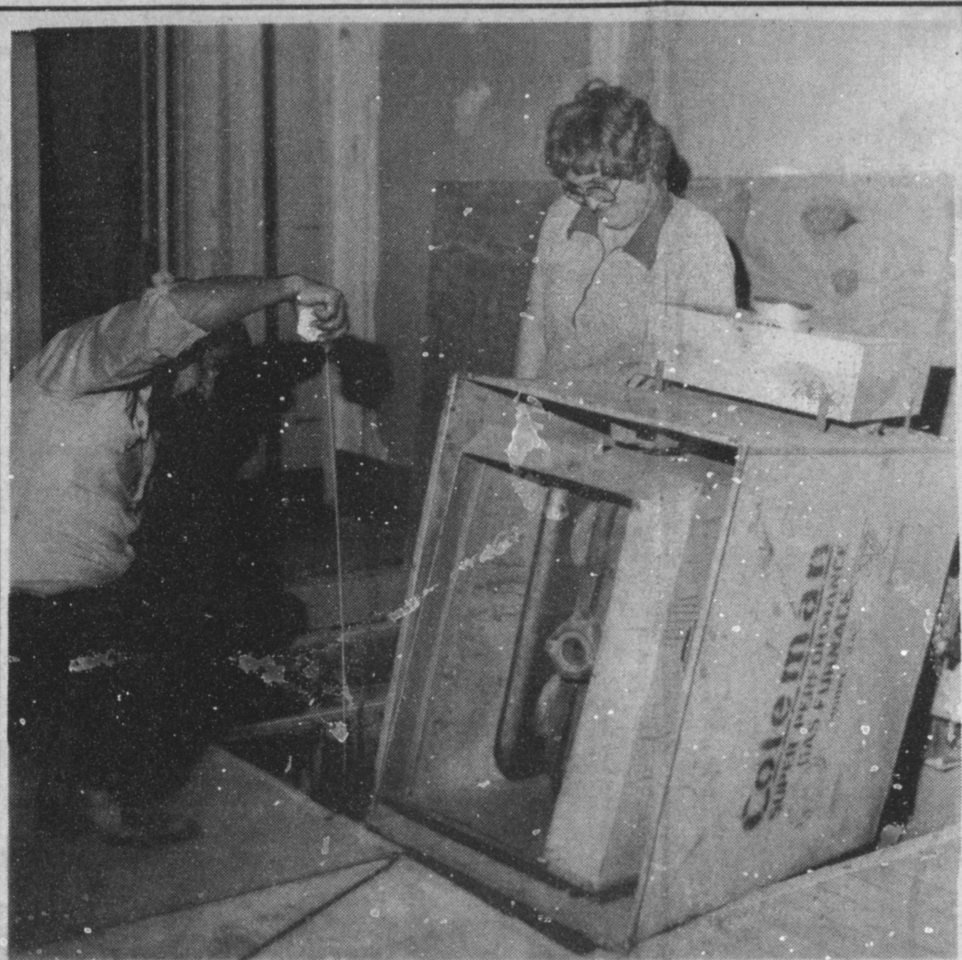
MEASURING FOR A TIGHT SPACE-Monday night, Ruben Leal, who has done a lot of volunteer work helping renovate the Girl Scout Little House, showed Nelda Merriott, Girl Scout Committee chairman, how a furnace will fit in the large meeting room of the Scout House. Although funds for renovation are low, the Girl Scouts are optimistic enough to believe more funds will be donated to help complete the renovations. Because of a limitation of funds, the renovation project has been slower than initially planned. But, because of volunteer work by many, many people, it continues to be an ongoing project.
