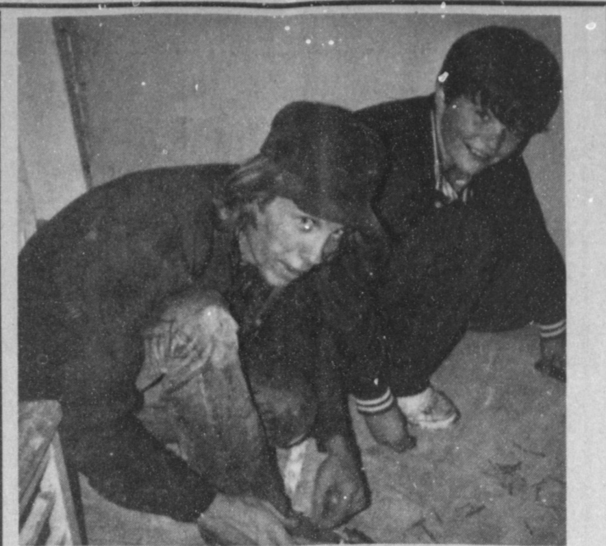
EVERYBODY VOLUNTEERS --Greg Williams, left, and Kalam Puckett are two of the volunteers helping with renovations at the Girl Scout Little House. Williams is volunteering his services, as well as Boy Scout Kalam. Also helping at this time are Larry Puckett, Kalam's father; mother, Cheryl Puckett and daughter, Kayna, a Daisy Scout.
