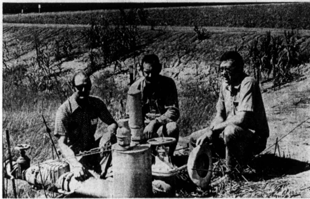
TAILWATER PIT — Excess irrigation water on Roger Dawdy's farm west of Floydada flows into this tailwater pit and is recycled back onto the field through an underground pipeline system. Jon LaBaume, district conservationist, Joe Platt, soil conservationist, and Roger Dawdy (l to r) examine the electric pump motor that regulates the system. (Staff Photo)
