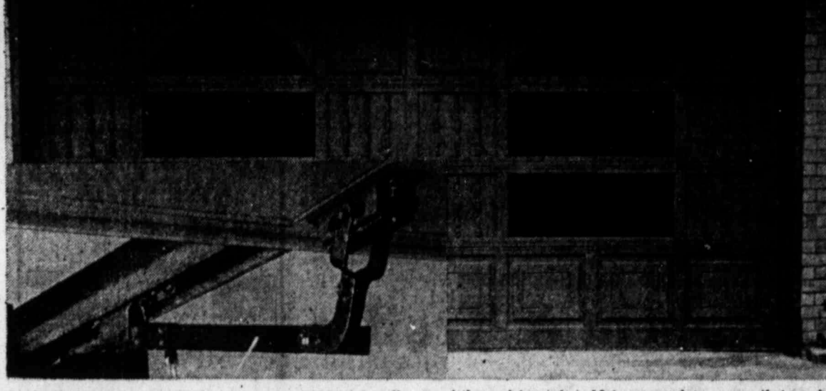
MODERN AND AVAILABLE — Shown is a Lubbock installation of an overhead automatic door (note its attractiveness) and the acclaimed Auto-Mate garage door opener that can be "a lift in your own situation," thanks to Overhead Door Co.
