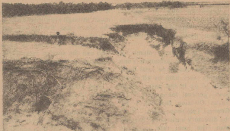
UNCONTROLLED WATER runoff on the M.B. Wardlow farm west of Robert Lee caused this serious gully and soil erosion problem.
