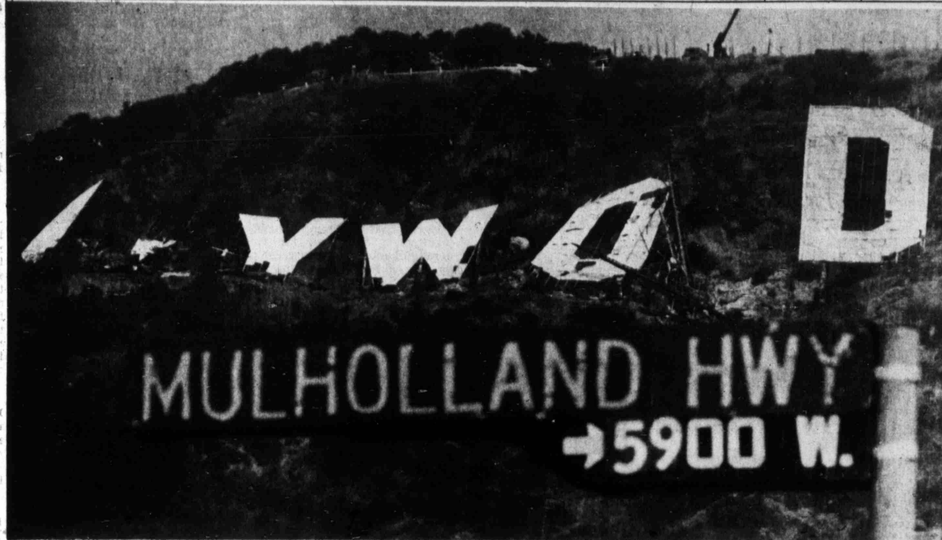
WORKMEN PREPARE to take down the "D" telephone poles and plywood, has succumbed by a new Hollywood sign financed by several letter of the Hollywood sign, from Mt. Lee in Los Angeles. The old sign, made from to the ravages of 55 years. It will be replaced recent fund-raising projects. (AP Laserphoto)
