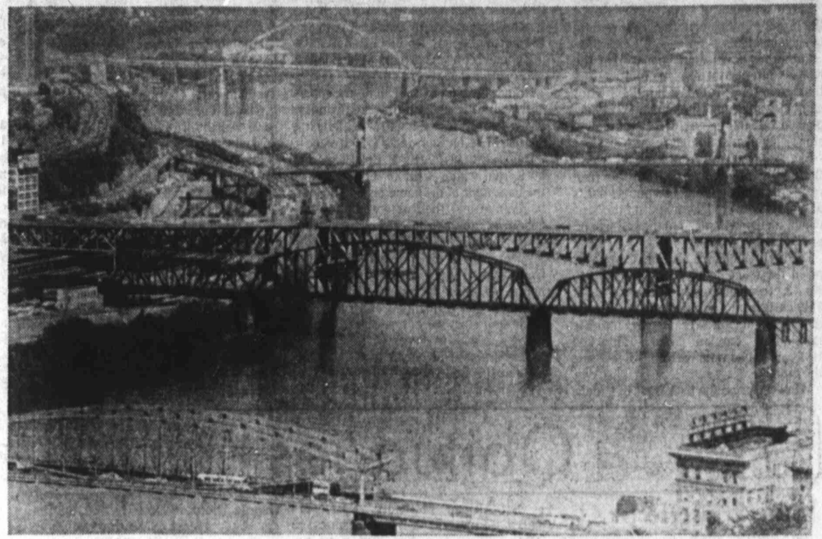
PITTSBURGH BRIDGES FALLING DOWN — These bridges, spanning the Monongahela River, are among the 1,800 serving Pittsburgh and surrounding Allegheny County that are worrying local officials. The spans average 50 years of age and are beginning to fall apart at an alarming rate. (AP Laserphoto)
