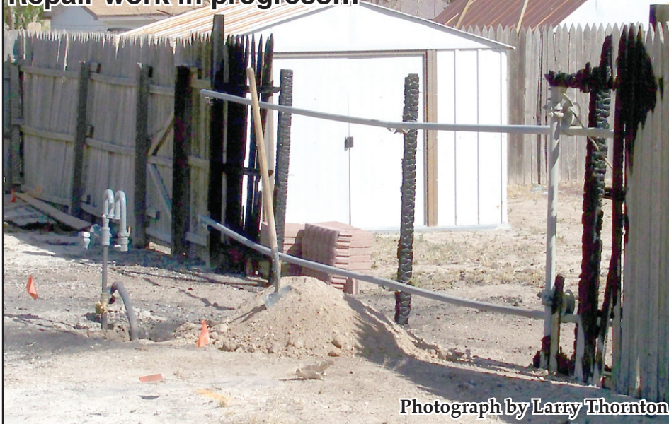
Repair work in progress...
