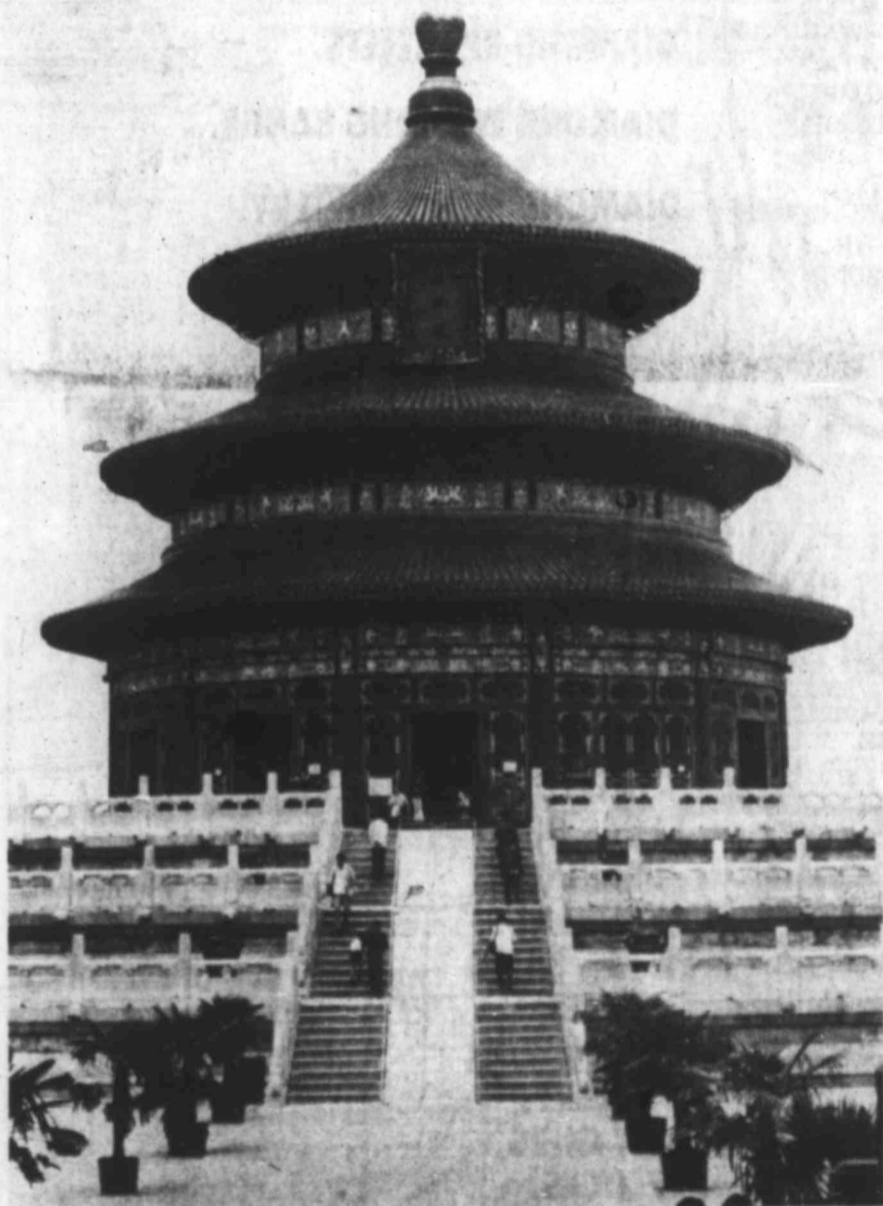
The Temple of Heaven in Peking was built during the Ming Dynasty as a place where the emperor could contemplate heavenly peace. A remarkable structure architecturally, the inside is expansive and open and one can see up the three-tiered roof to a five-toed dragon, the emperor's symbol, at the pinnacle.
