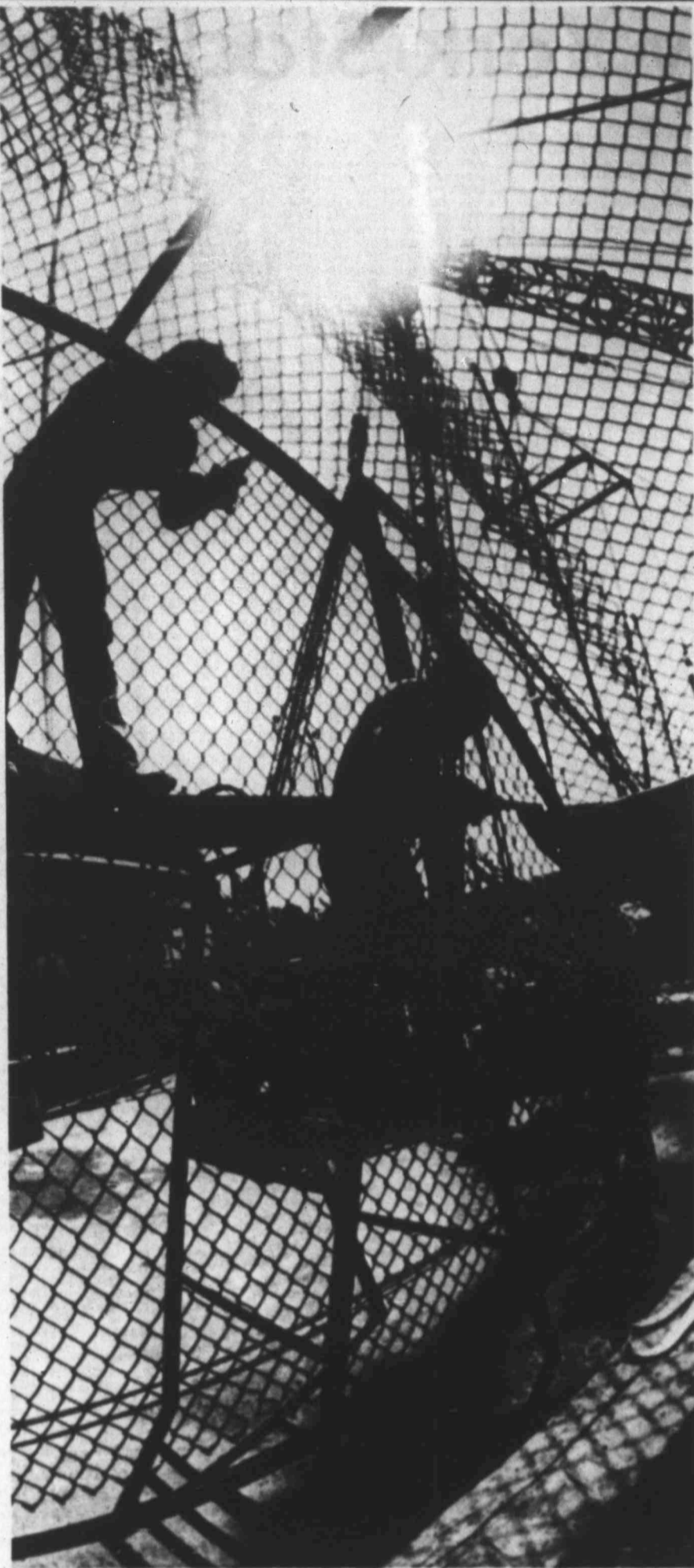
WORKMEN construct a cage at Dereckter shipyards in Mamaroneck, N.Y. Attached to floats and powered by twin outboard engines, the cage will form a protective barrier about long distance swimmer Diana Nyad when she attempts to swim from Havana, Cuba, to Florida. (AP Laserphoto)
