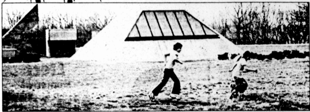
Terraset is covered with dirt. Up on the rooftop kids play. The dirt makes good insulation. It helps store the heat during the winter and the coolness during the summer. The school was built by shaving off the top of a hill, building a school and putting the dirt back. Terraset uses electricity, too. The electricity operates the machines that change the solar heat into energy. A skylight is in the background.
