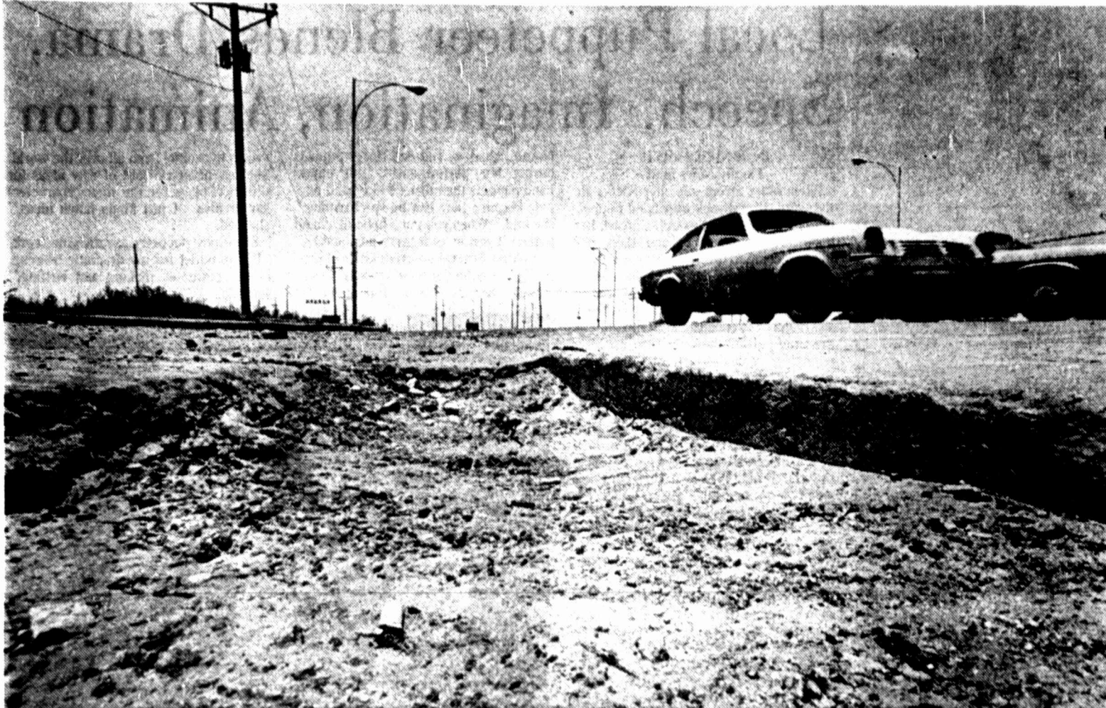
POTHOLES APLENTY — Lubbock motorists driving on Belmont Drive near the Brownfield Highway in West Lubbock are faced with numerous potholes as obstacles. The potholes began showing up following the heavy rains in late May. (Staff Photo by Milton Adams)
