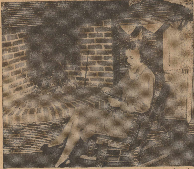
PIGEON COVE, MASS.—Well, almost nothing, except that the pretty lassie above is sitting on a paper chair, reading by the light from a paper lamp, and of all things, warming herself in front of a paper fireplace. Hard to believe, but true. The entire house is made of old newspapers tightly rolled and coated with Waterspar Varnish, which makes the papers both water-repellent and weather proof. It's a unique answer to the housing shortage.
