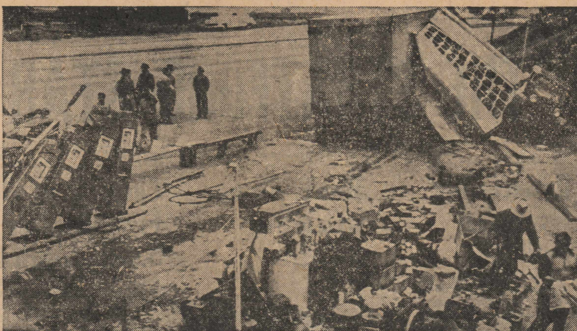
BRISBANE, CALIF.—(Soundphoto)—Tilted gas pumps and mass of debris are all that is left of steel-frame gas station here after it was hurled off its foundation and carried 20 feet when a huge 18-wheel truck-trailer veered off Bayshore highway and smashed through it. John Vincoquerra, 24, San Jose Calif., the truck driver, said two automobiles in front of him suddenly stopped directly in his path. He applied airbrakes, but they failed, and he swerved to avoid hitting the cars. The truck plunged across curbing and into gas station, carrying it with it before coming to rest (rear) against hill.
