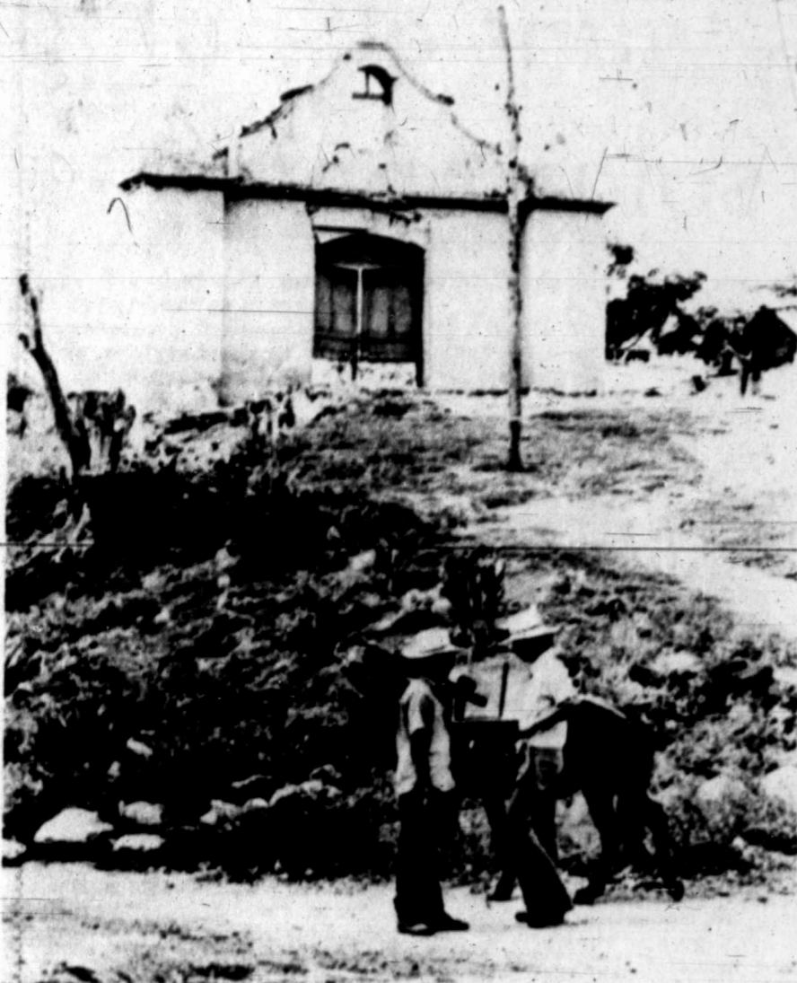
Only the front wall and doors of a village church remain standing after one of Guatemala's numerous quakes struck the area. Reconstruction of the devastated areas, particularly those hard hit by the 1976 quake, is under way with the help of the World Food Program's food-for-work project.
