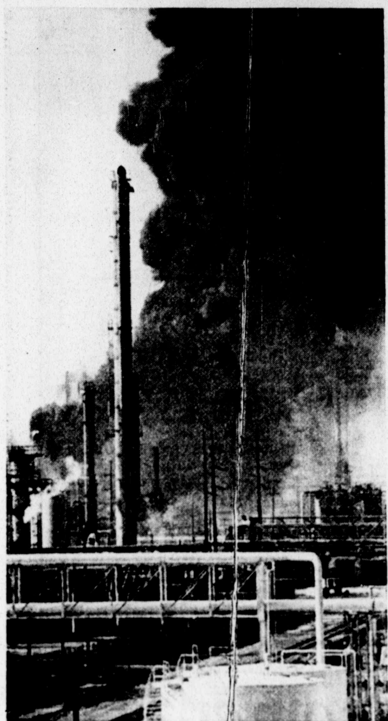
CONTINUES BURNING — The Texas City refinery fire is shown as it continues to burn late Tuesday. Several explosions rocked the plant early Tuesday morning. Fire departments from many towns in southeast Texas were called in to help fight the Texas City disaster. (AP Laserphoto)
