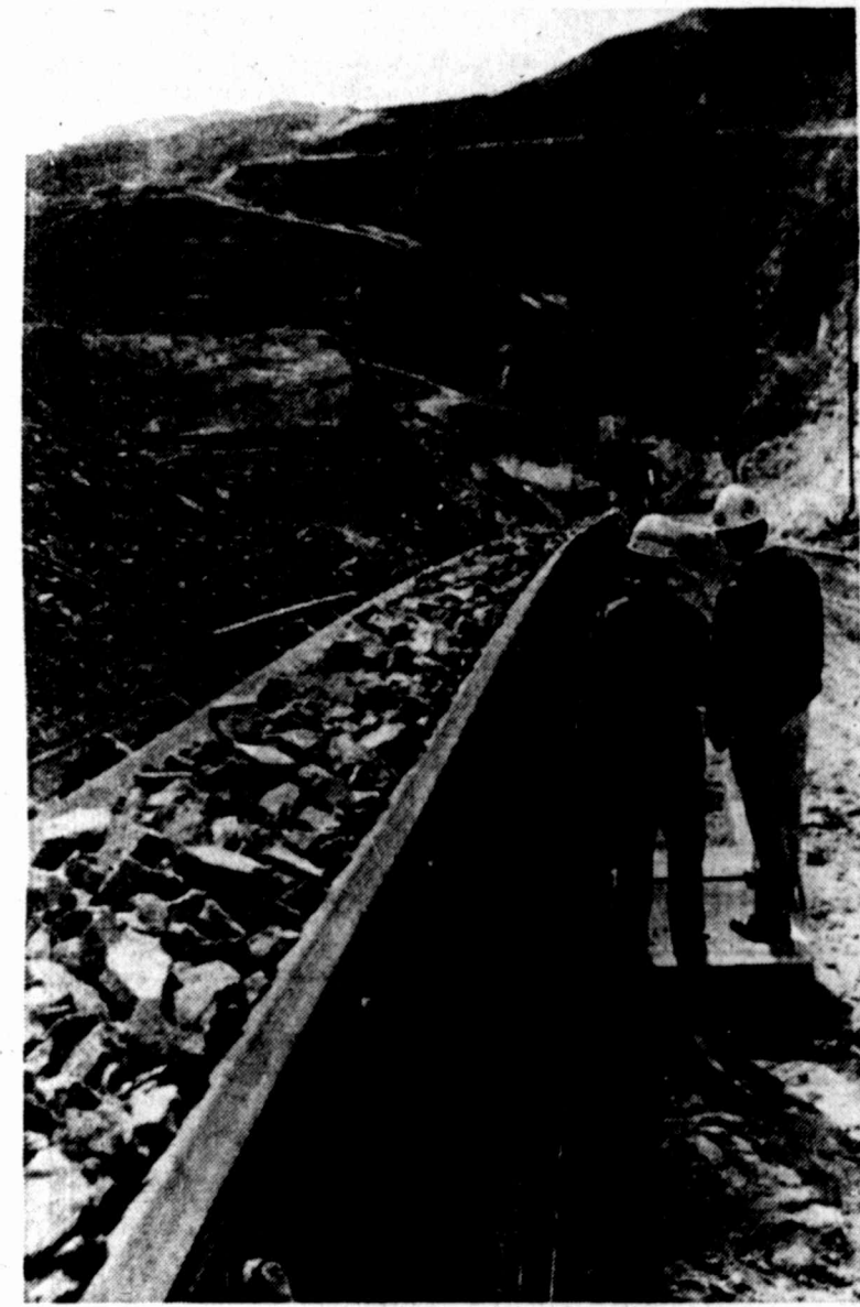
FUEL-SAVER — This giant steel cable belt, made by Goodyear as part of a conveyor system at a Tucson copper mine, does the job of a dozen 120-ton trucks. The belt can move up to 6,400 tons of ore an hour and will save $31 million in fuel costs over the next 10 years. (AP Laserphoto)
