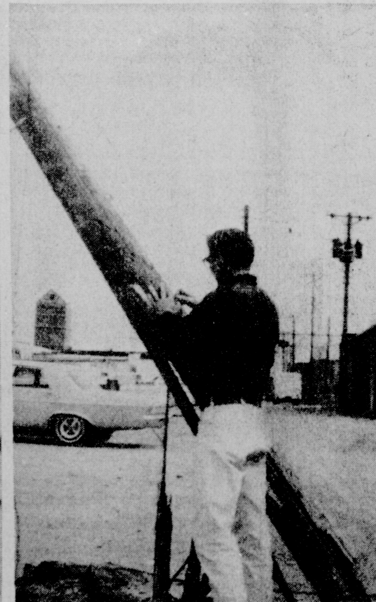
equipment installer for General Telephone, examines the broken cable, and at right, he looks over a snapped-off cable pole. (Journal Photos)
