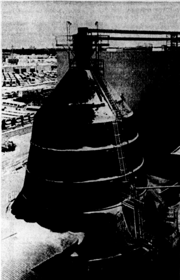
ENERGY SAVER—Stretching coal supplies at GMC Truck & Coach plants in Pontiac, Mich., is a unique refuse-burning system which mixes scrap wood, cardboard and paper with coal to fuel steam power boilers. Introduced in late 1975 as part of the company's energy conservation program, the system utilizes approximately 48,000 tons of industrial scrap yearly to save about 30,000 tons of coal.
