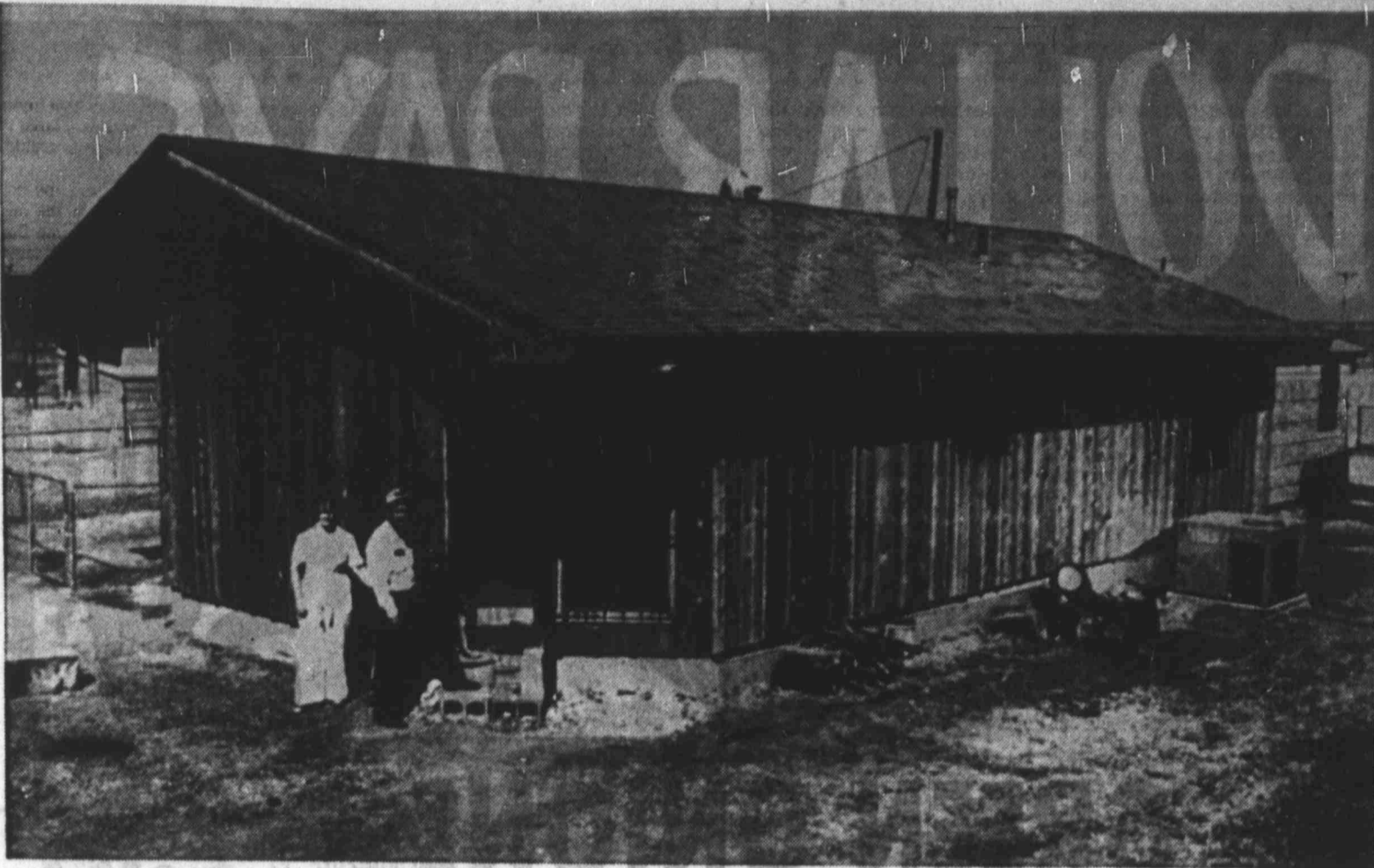
A HOUSE DIVIDED — Mr. and Mrs. Robert Groth live in a house divided — that is, ready to be divided when they retire. They designed and built this home in Laverne, Okla., so that it can be divided in the middle and moved 300 miles to the lake property they plan to retire on. (AP Laserphoto)
