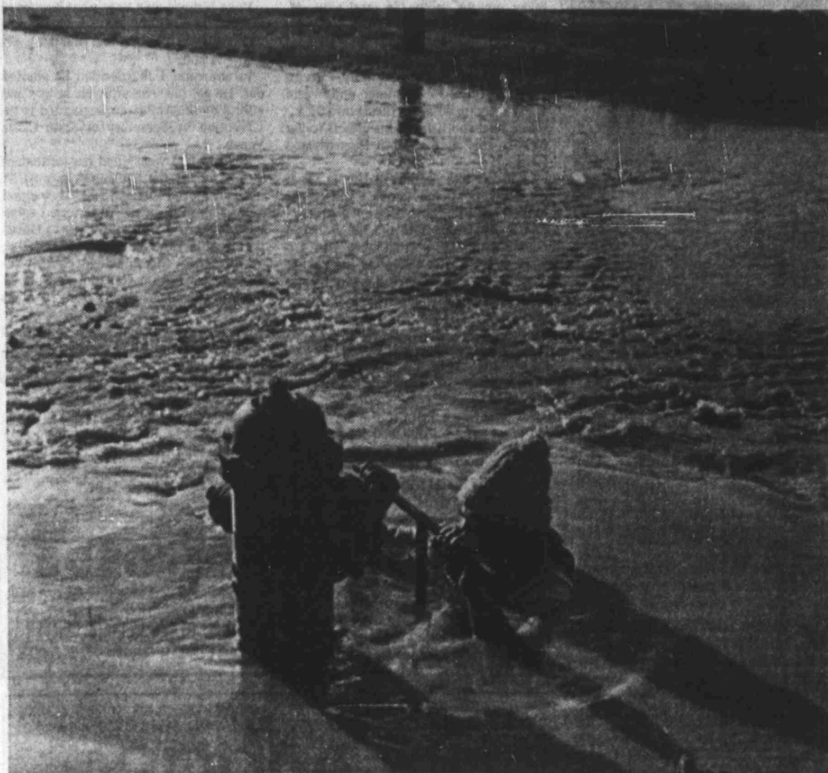
HOW HIGH'S THE WATER, MOMMA? — When Lawton, Okla., city water department worker Doug Spencer was called to turn off a fire hydrant Wednesday afternoon, he didn't dream he'd wind up in water up to his stocking cap. The plug began its unscheduled eruption after a car hit it. (AP Laser-photo)
