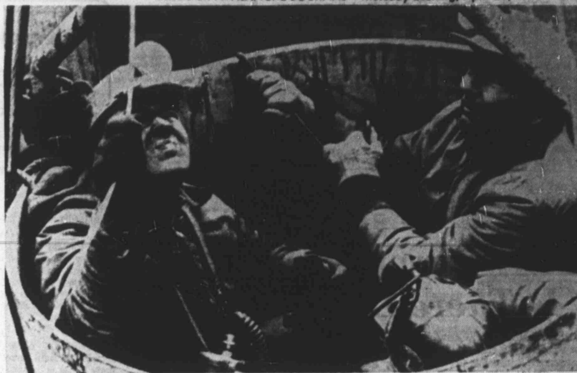
DECADE OF RECOVERY EFFORTS CEASE — Three miners are listed by bucket from the No. 9 mine near Farmington, W. Va., on Nov. 20, 1968, after explosions ripped through the shafts and killed 78 miners. They were among the first to be rescued, and 19 men were never found. After ten years and $11 million in recovery efforts, the Consolidation Coal Co. has decided to cease their search, against the wishes of the dead men's widows. (AP Laserphoto)
