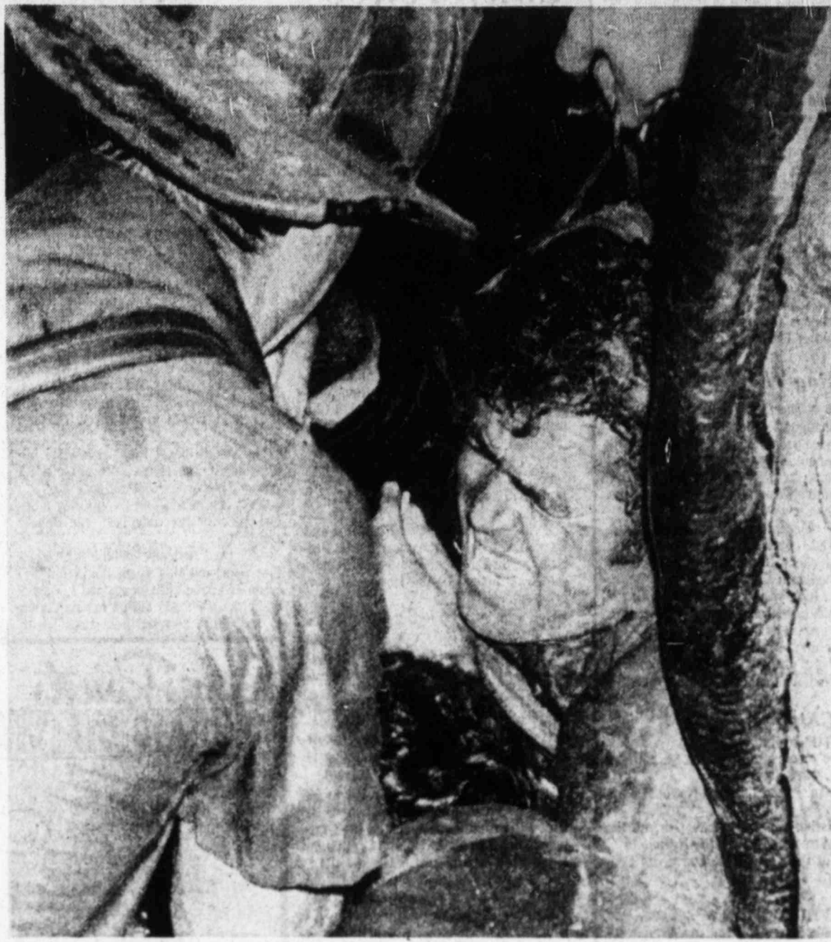
WORKER RESCUED — Construction worker Vito Tautonico, 46, of Flushing, N.Y., grimaces in pain as other crew members free him from mud and water in a sewer excavation. He was trapped when the walls collapsed. (AP Laserphoto)
