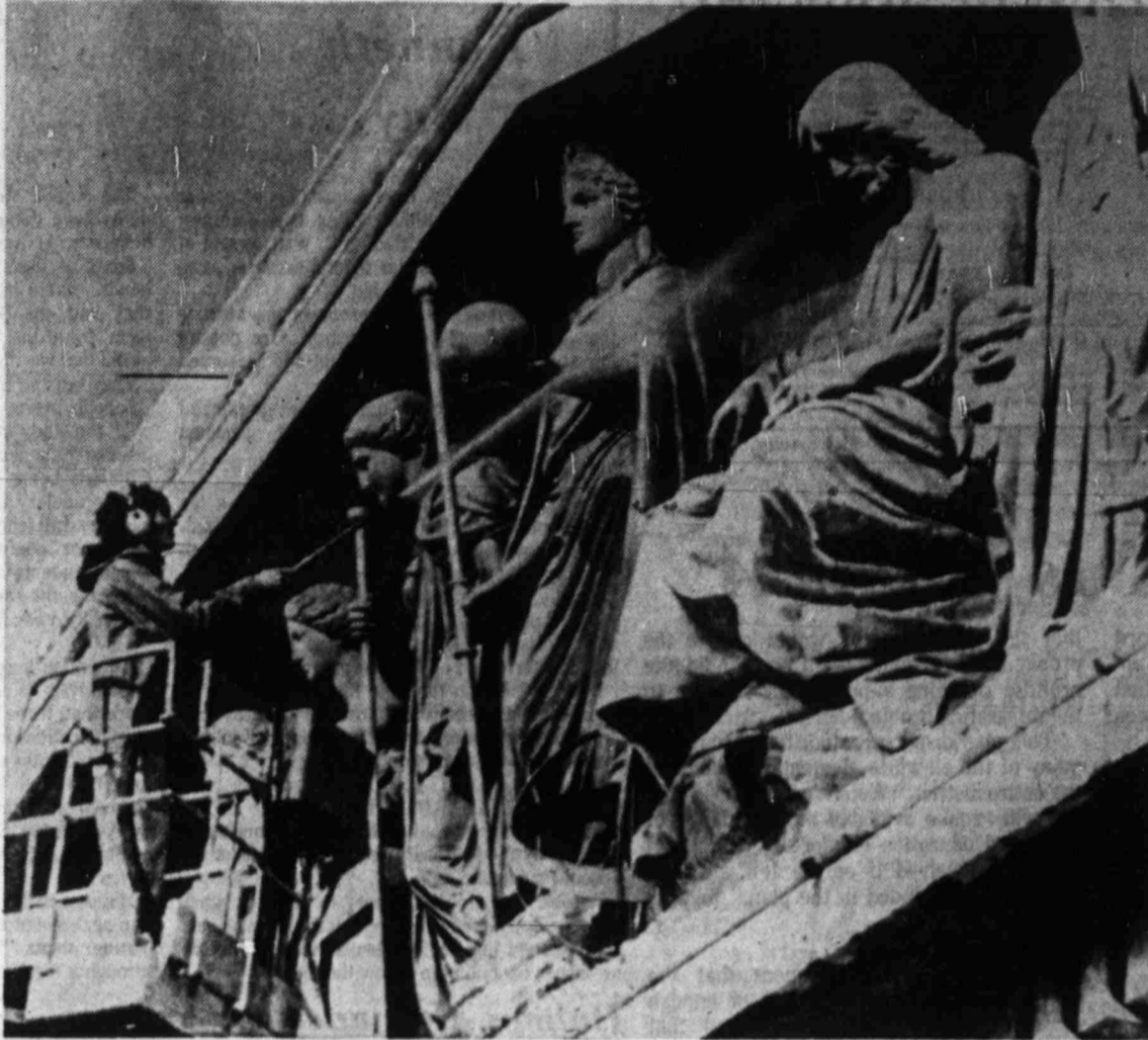
BIG CLEAN-UP — A cleaning company worker turns a high pressure hose onto statues over the main entrance of the British Museum in London during a massive clean-up operation of the building. The company is using hydraulic lifts in place of scaffolding, cutting the costs in half to $110,000 for the face-lift. (AP Laserphoto)
