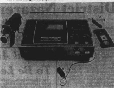
CREATORS OF OUR OWN CULTURE?-Technological developments, such as this RCA video cassette recorder, may provide greater individuality in our culture. Features include: 1. optional camera which allows production of home shows, 2. speed switch which allows up to four hours recording time, 3. remote pause control, 4. tape counter with memory, 5. electronic digital clock/timer for unattended recording, 6. optional microphone, 7. cassettes with four-hour recording capacity.
