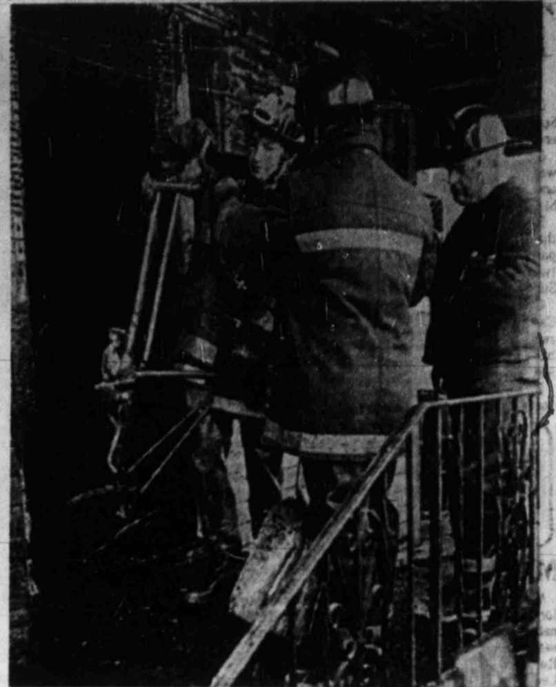
WHERE SEVEN DIED — Firemen remove the twisted remains of a bicycle from the charred doorway of a three-story apartment building Sunday morning in Lawrence, Mass., after a fire, which raged out of control for three hours Sunday morning, killed seven persons, including five children, in a third-floor apartment. (AP Laserphoto)
