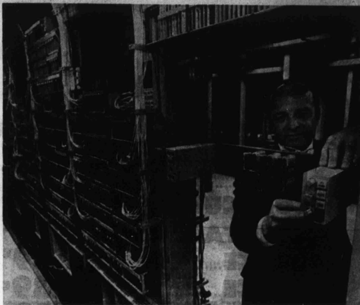
SUPER SWITCHER — Richard E. Pitts, a regional manager for American Telephone and Telegraph Company, demonstrated a new telephone switching system in Washington this week. This system, called a "super switcher," has the capacity to handle 550,000 long distance calls an hour. Pitts stated that this system will speed up the time it takes to make long distance calls as well as cut the cost of service. (AP Laserphoto)
