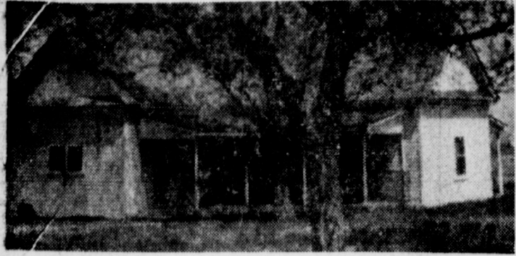
LANDMARK SELLS — This old cookhouse of the Muleshoe Ranch is included in property sold to Medlock Co., Lubbock, this past week. However the building, a Historical Society plaque-bearer, will be retained and improved, the new owner says. (Journal Photo)
